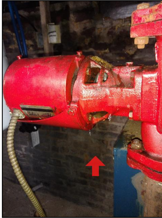
Leaking pump
